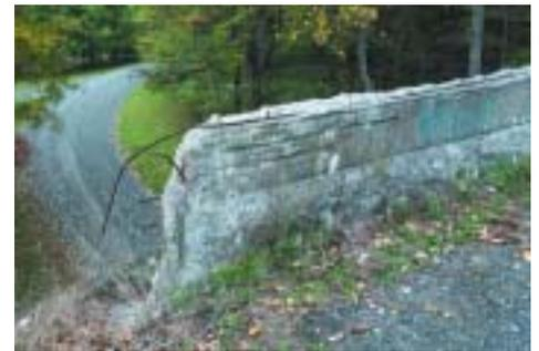
Figure 1. Exposed steel reinforcement is result of freeze-thaw damage to concrete bridge.
